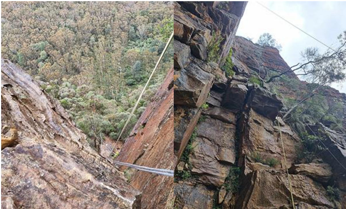
Photos of the incident site.
